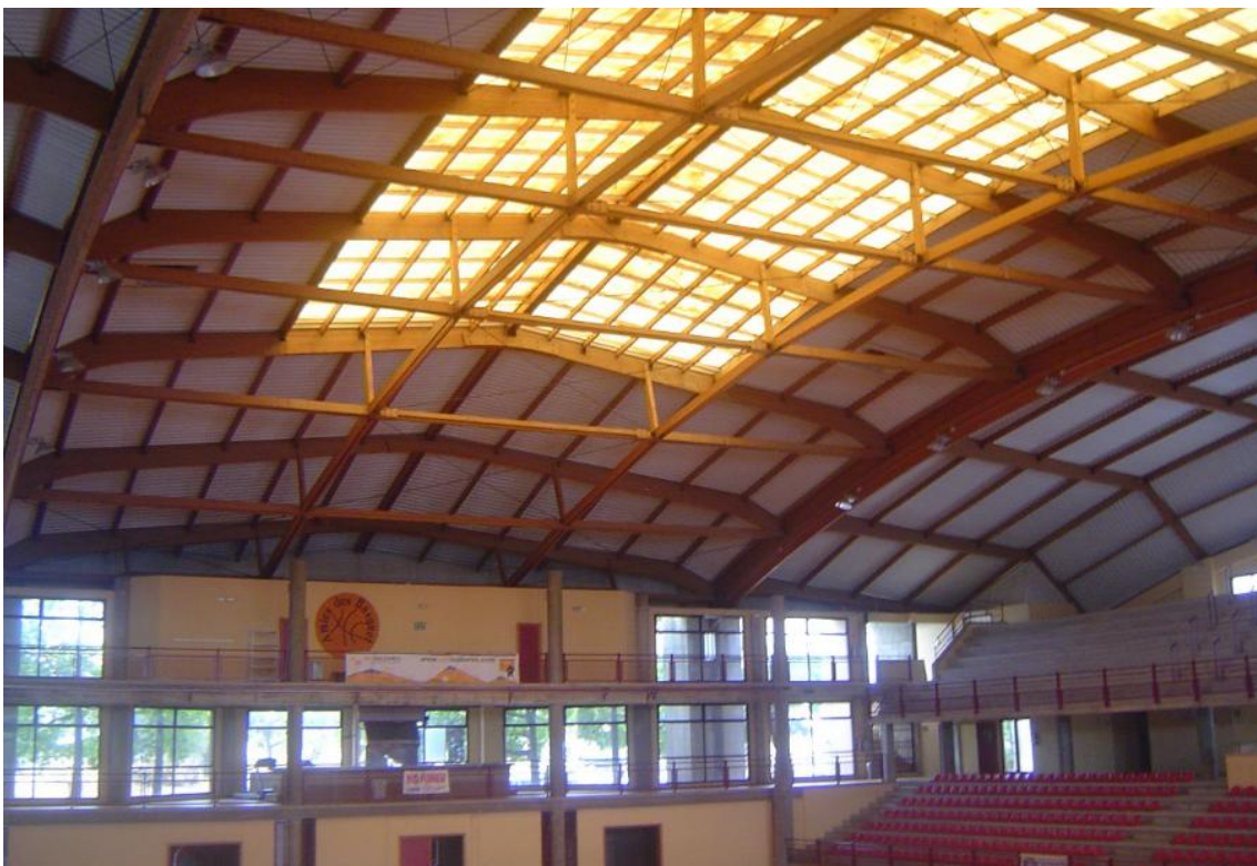
Vista general de la coberta i lucernari
